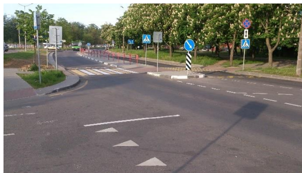
Fig. 2. The typical example of the street-refuge's installation in Minsk, Belarus.
