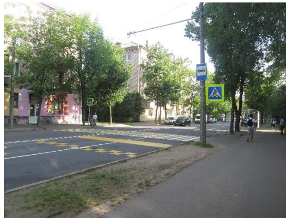
Fig. 1. The typical example of the hump's installation in Minsk, Belarus.
