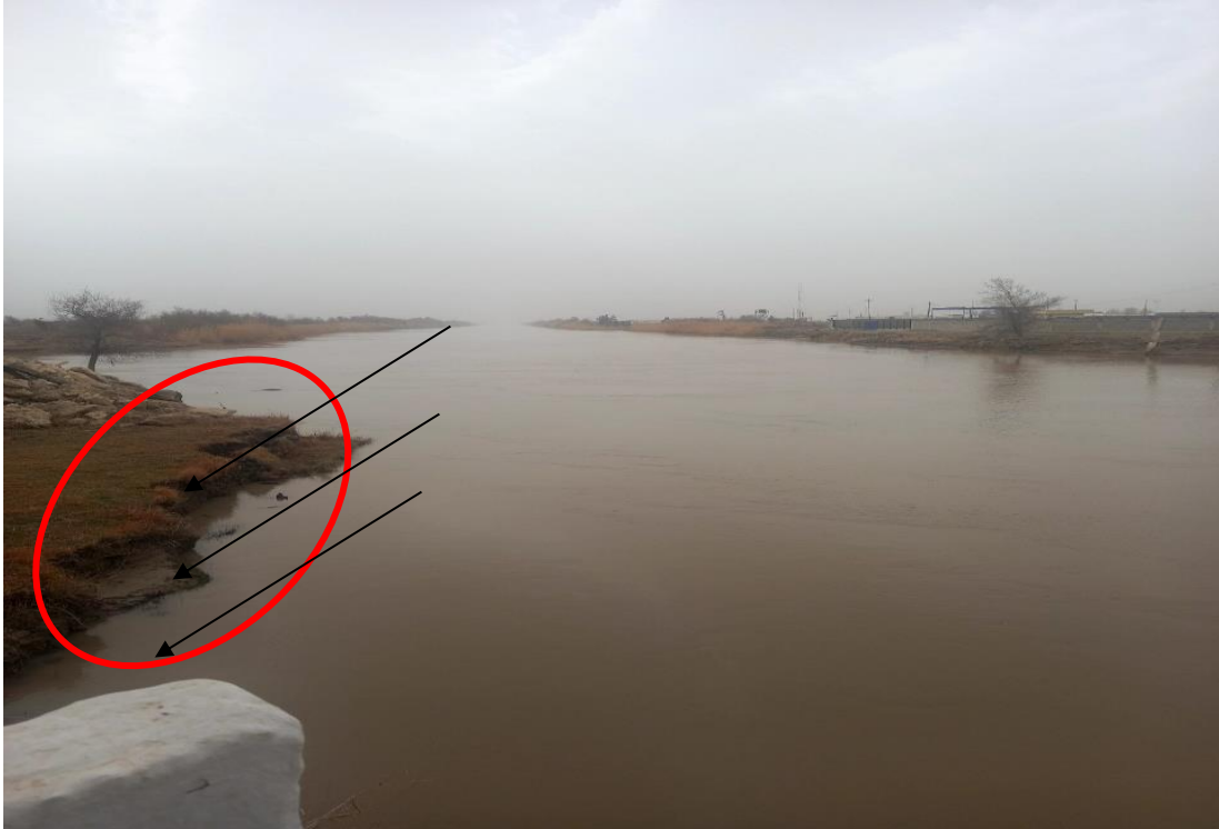
1.1-picture The state of washing of the banks of the building's supply channel
