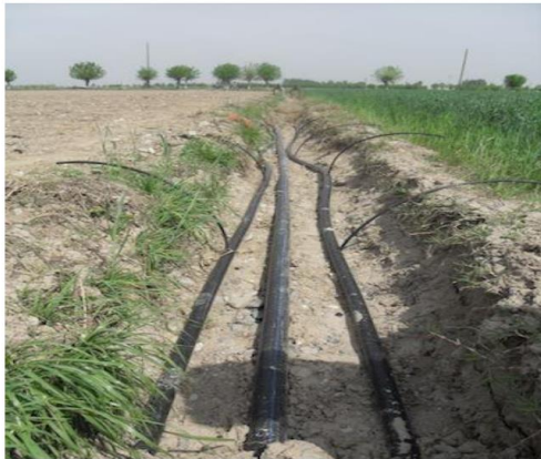
Fig. 1 The process of laying drip irrigation lines in the field in Namangan
