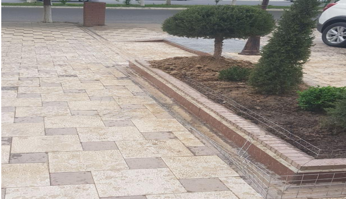
Figure 5. The process of building a gabion on Sebzor street
