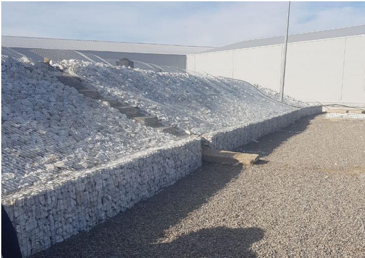
Figure 3.4. The finished state of gabions at "OOO BAKAN TEX"
