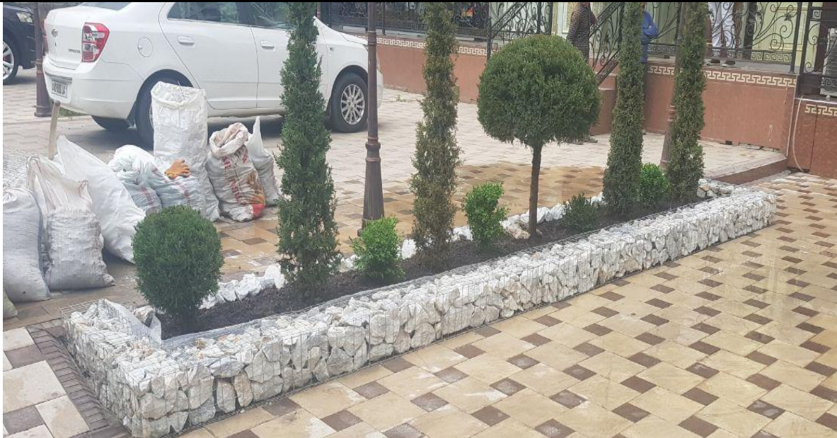
Figure 7. Building a gabion on Sebzor Street
